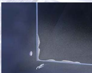
**E.** As the process continues, AEROSEAL's adhesive continues to build up on edges of holes...
